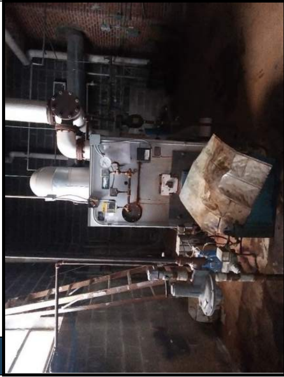
6 Hard joint tested positive for asbestos (65% chrysotile).
