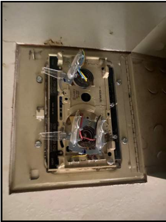
13 Mercury thermostat in the cafeteria.
