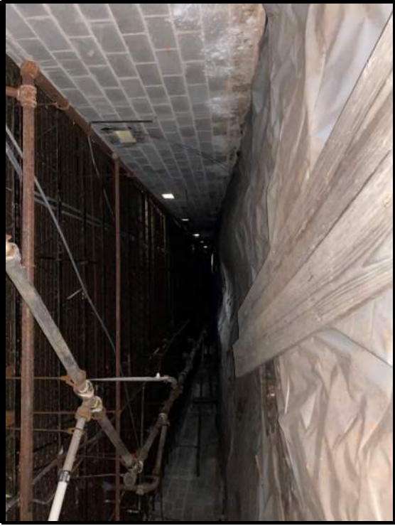
12 General view of crawlspace.
