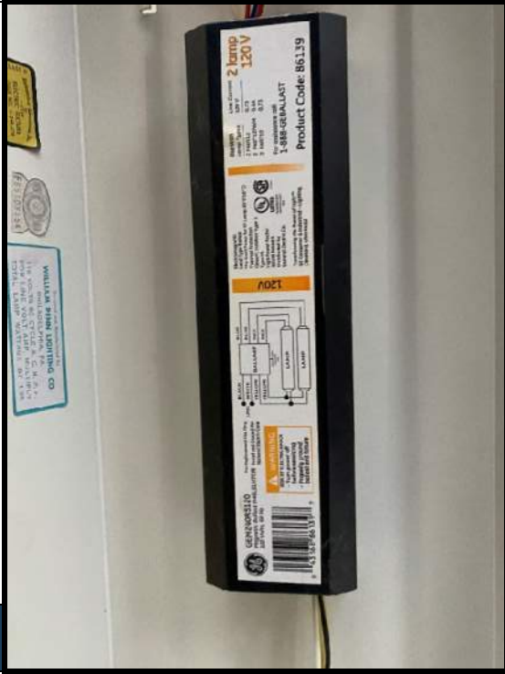
14 Ballast labeled no PCBs.
