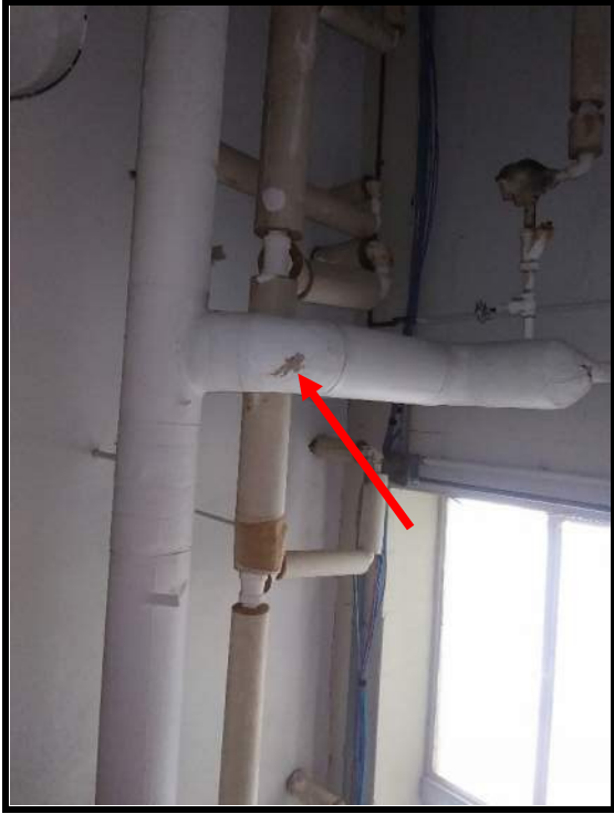
6 Hard joint tested positive for asbestos (65% chrysotile).
