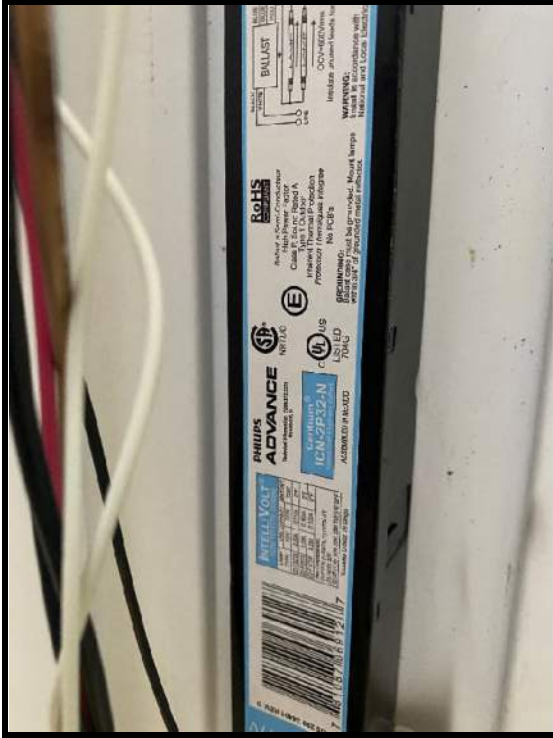
14 Ballast labeled no PCBs.
