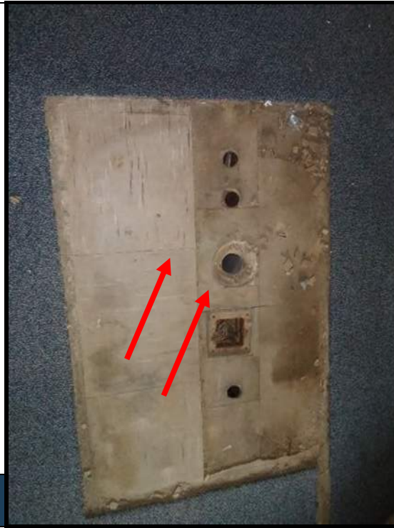
3 12-inch dark tan vinyl floor tile and black mastic and 9-inch brown vinyl floor tile and mastic tested positive for asbestos (3% chrysotile).
