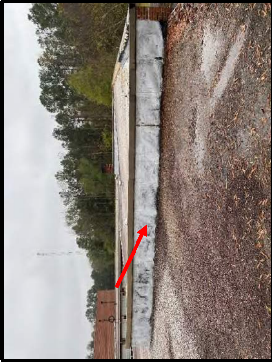
11 Silver sealant on parapet walls tested (<1% chrysotile) PLM analysis and no asbestos detected by TEM.
